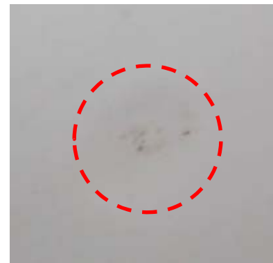
Impact Damage Outboard View
